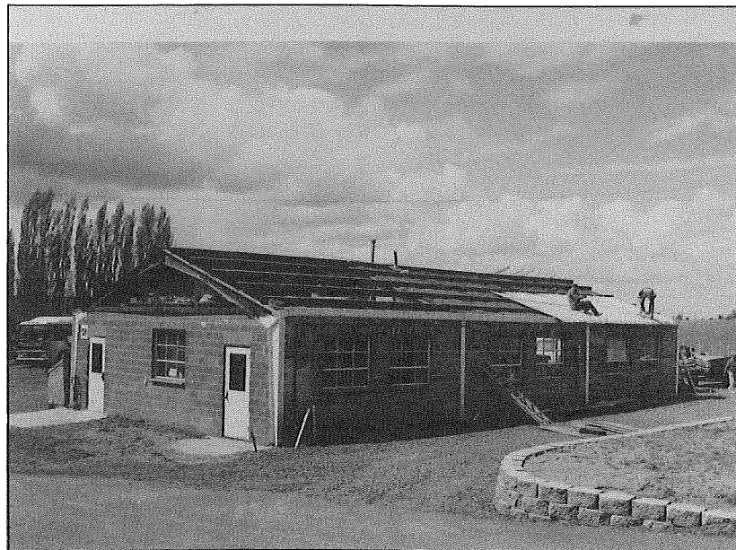
Another big improvement appears on campus. The old metal roof is taken off the maintenance shop in preparation for an asphalt-shingle replacement. Although not a regular Maranatha project, most of the work was done by volunteers, many of them Maranatha regulars.
